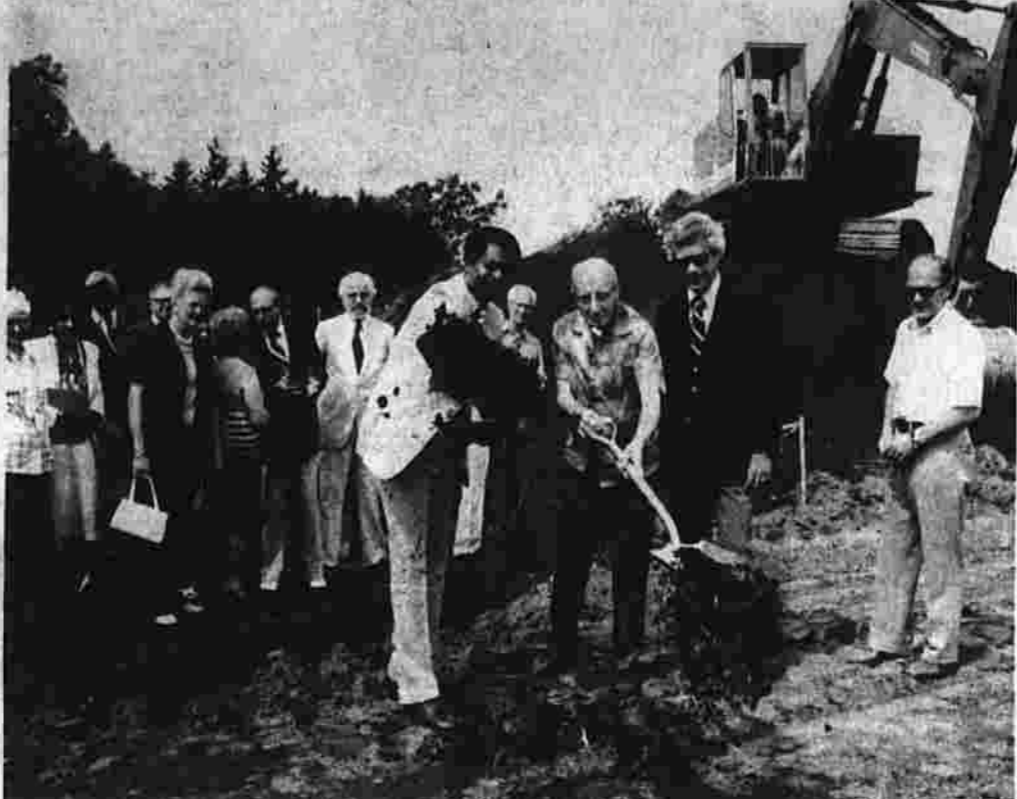
Ground broken for housing project. State and local officials gathered this morning at the site of Manchester's new housing for the elderly project on Spencer St.
